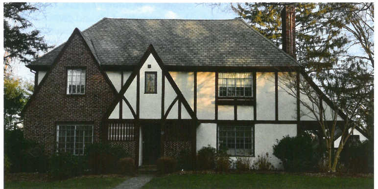
A larger Tudor Revival home, with two prominent, steep, front-facing gables, stucco and brick wall materials, and decorative half-timbering.
