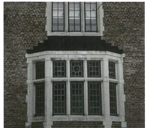
From left: Detail from a Tudor Revival home, including diamond-shaped window panes; decorative half timbering; four chimney pots; and some Craftsman-style brackets under the peak of the gable. Many Tudor Revival homes incorporate a mixture of interesting brick patterns. An elaborate bay window with leaded glass and stone window surrounds.
