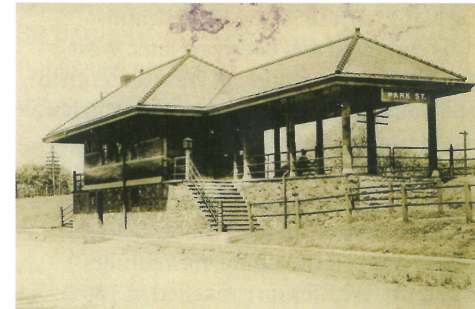
Park St./Watchung Ave. Station ca. 1910
