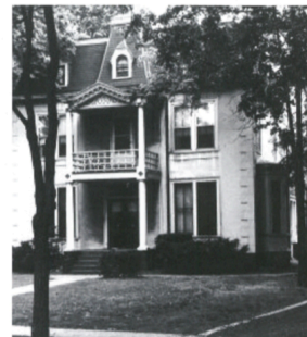
48 Walnut Crescent, the Lawrence Earle House, was built in approximately 1850.
